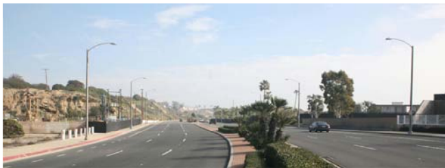
EXISTING VIEW FROM POINT A
