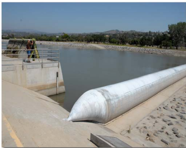
FIGURE 4-4 INFLATABLE DAM ON THE SANTA ANA RIVER
