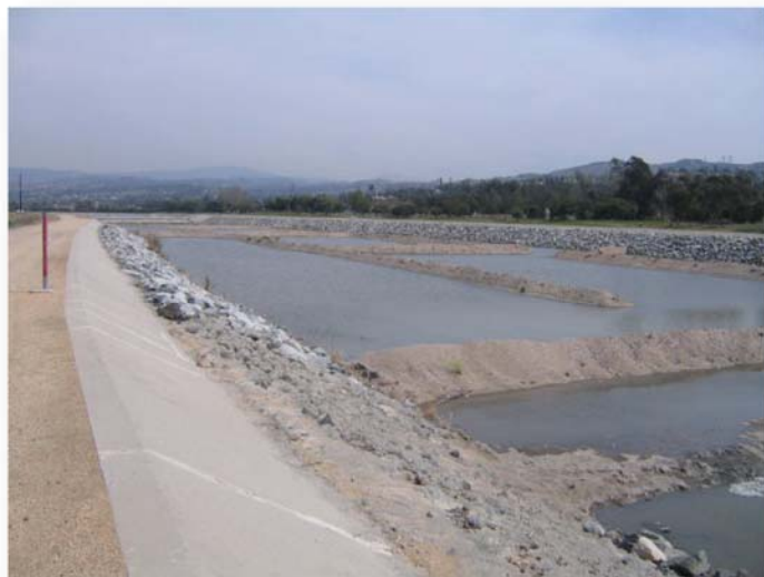
FIGURE 4-5 SAND LEVEES IN THE SANTA ANA RIVER
