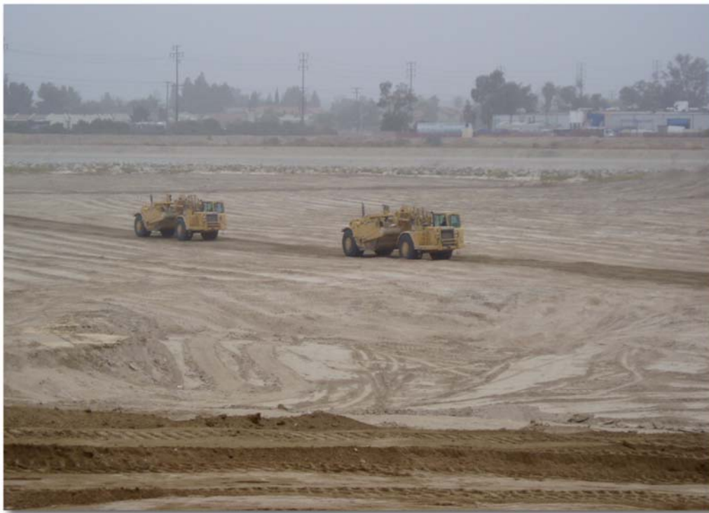
FIGURE 4-6 CLEANING OF RECHARGE BASINS
