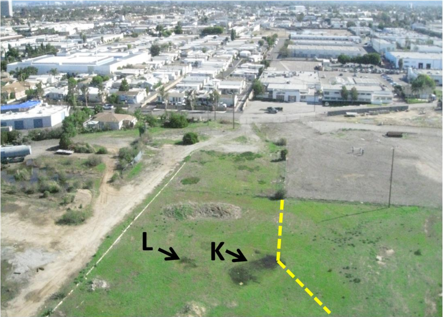
Figure 6 1/28/10 Looking towards east
