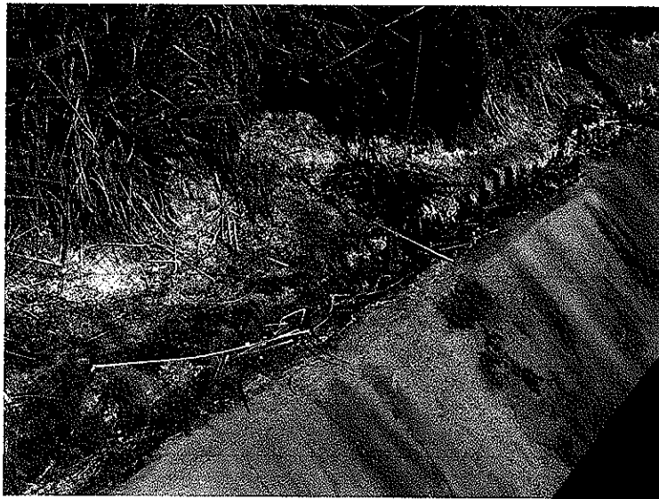
Figure 3. The slope above West Coast Highway also shows evidence of wetland conditions. This photo shows moist soils, a conspicuous salt crust, and apparent oxidation stains on the side of the concrete ditch, all indications that the groundwater seepage above Superior Avenue, shown in Figures 1 and 2, also occurs on the slope above West Coast Highway.
